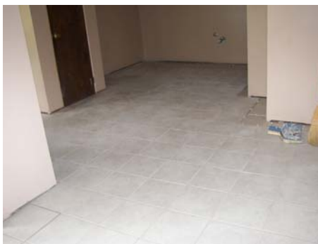
Job almost finished
