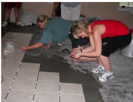
Laying tiles in living room
